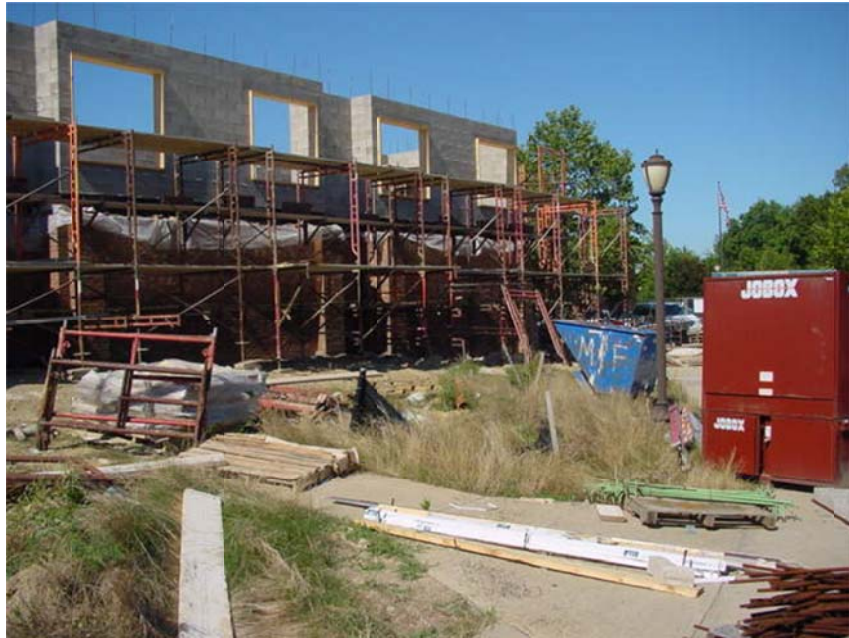
(Figure 5: Area B Masonry)
